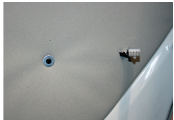
4b.4. Slowly screw the 3.9x16mm collar screw with 20mm dia. washer into the prepared drill hole for stabilization.
